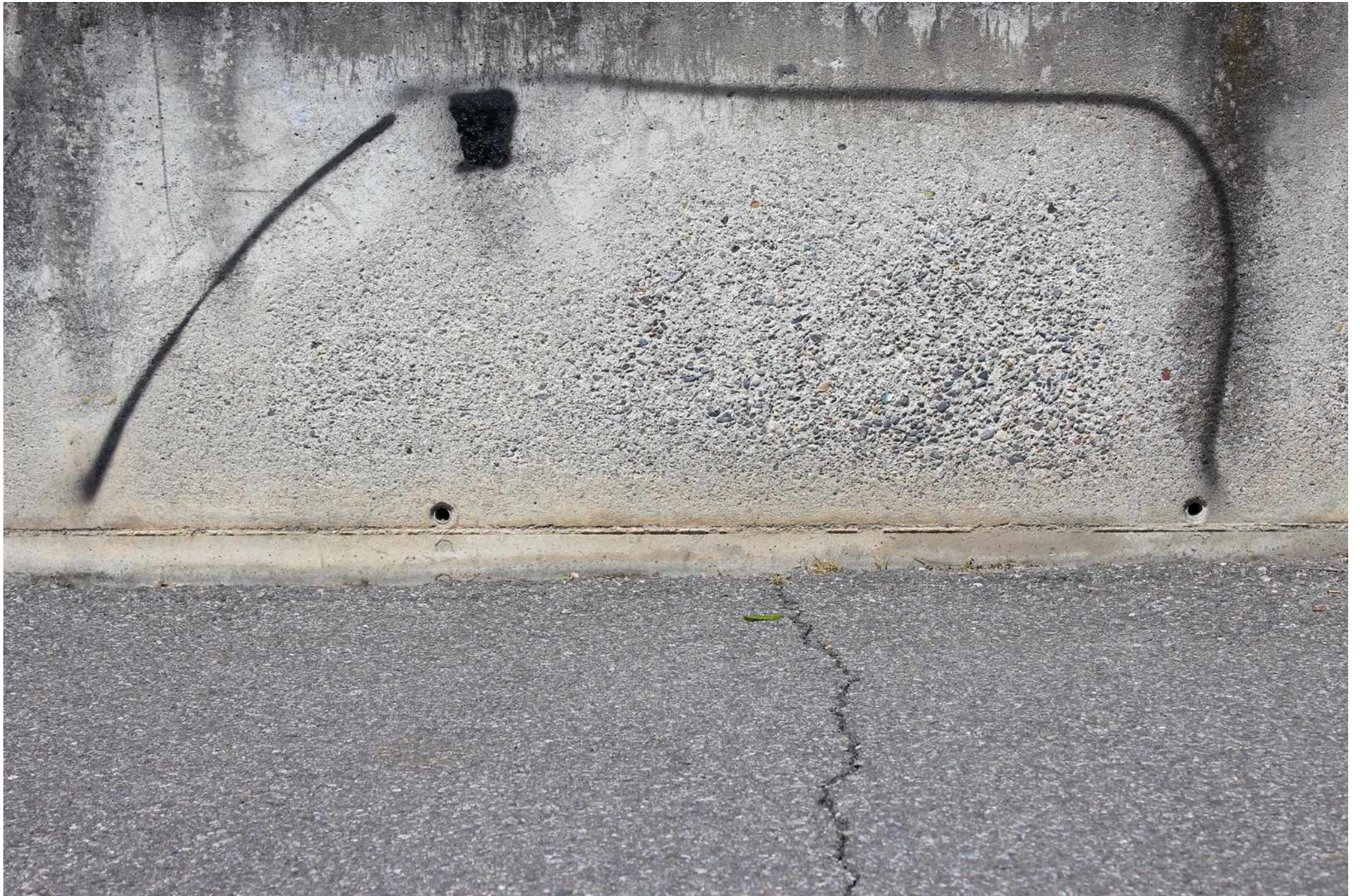
"D" intervention site specific, spray on wall
